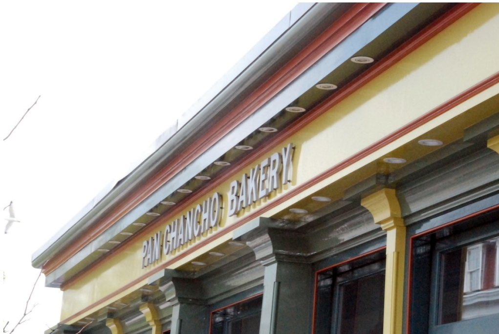
Multiple forms of lighting types and styles of downcast lighting that provides light to the storefront while limiting spillover.
