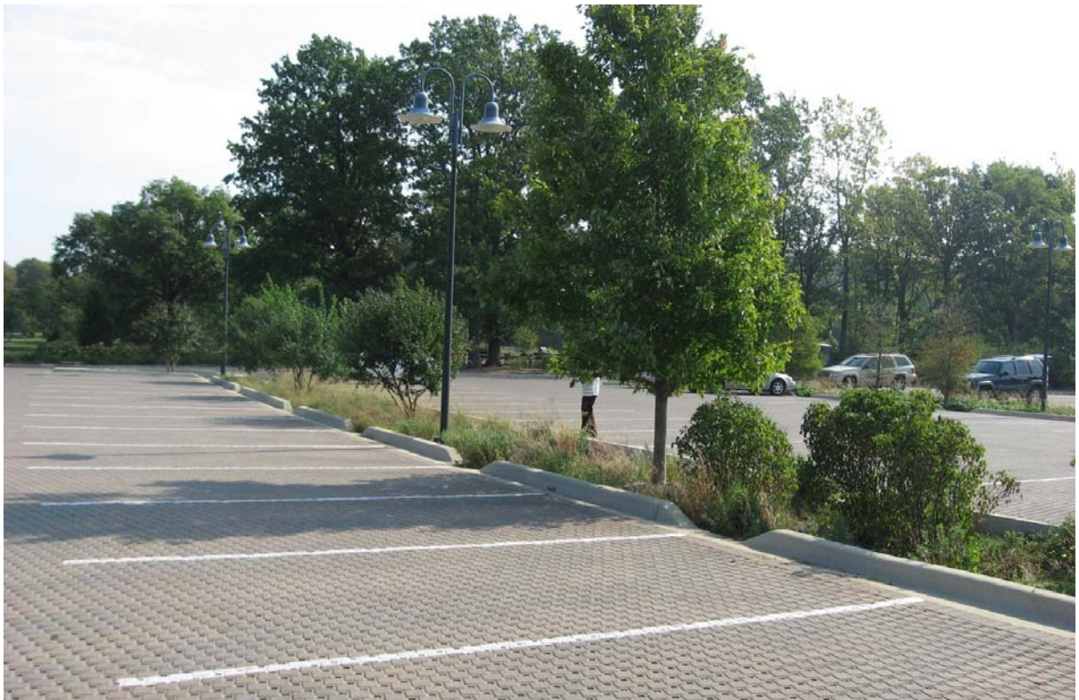
Trees within parking lots need sufficient space and appropriate subsurface conditions for roots to grow, such as this sustainable solution with storm water runoff.
