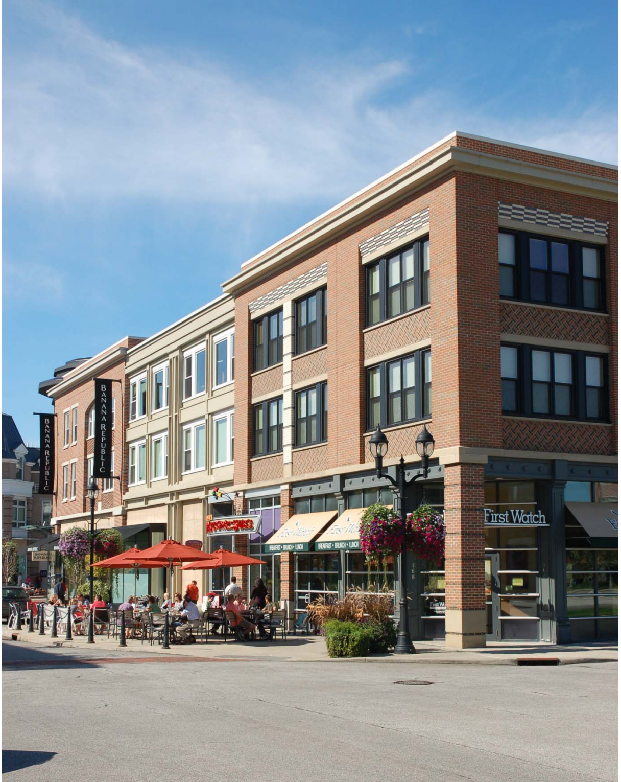
New multi-storey commercial development that follows good main street principles in terms of ground floor orientation with complementary upper storey articulation and materials in a traditional fashion.
