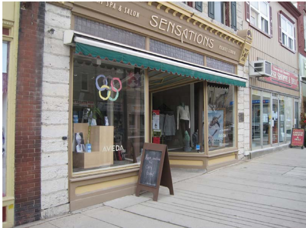
All the components that lead to a transparent façade at the pedestrian level: large glass panes, recessed entrance with glass, traditional commercial entrance door, and minimal window obstructions.
