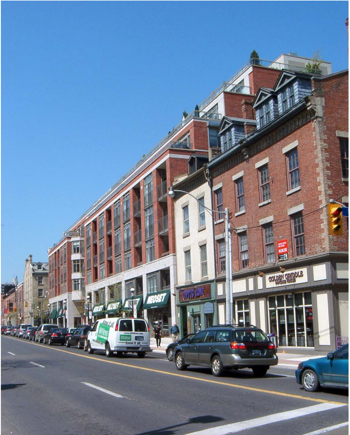
Development that steps the back the upper storeys to preserve the human scale and ground orientation of the streetscape.
