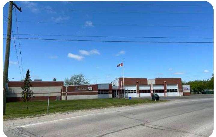
Thorold Fire Station 2 and Emergency Services, View looking west
