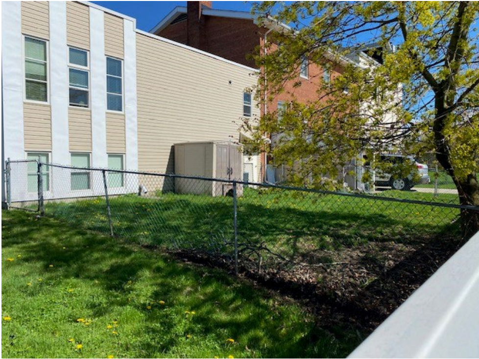
Figure 3: Existing Street View from West Street South looking south
