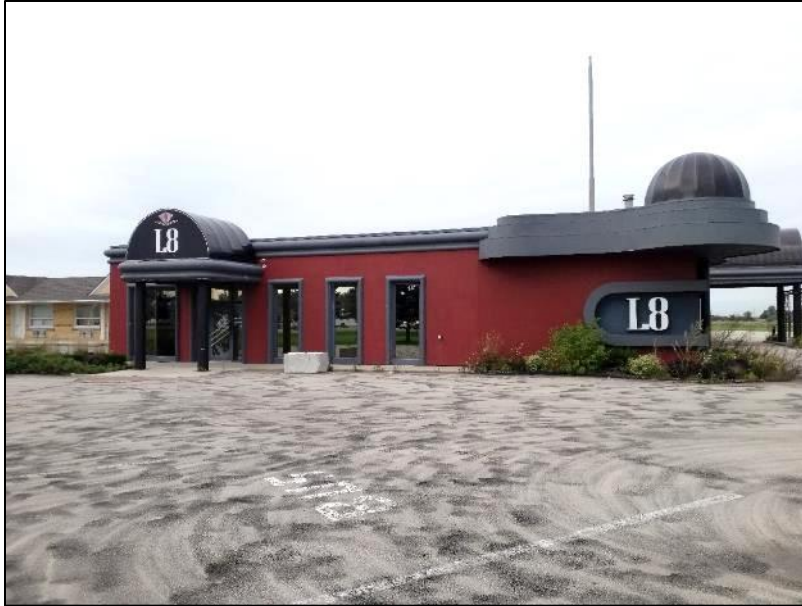
Image 3: Former nightclub in the east wing of the former motel complex.
