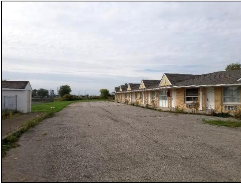
Image 1: Former motel complex with an asphalt parking area facing northwest.
