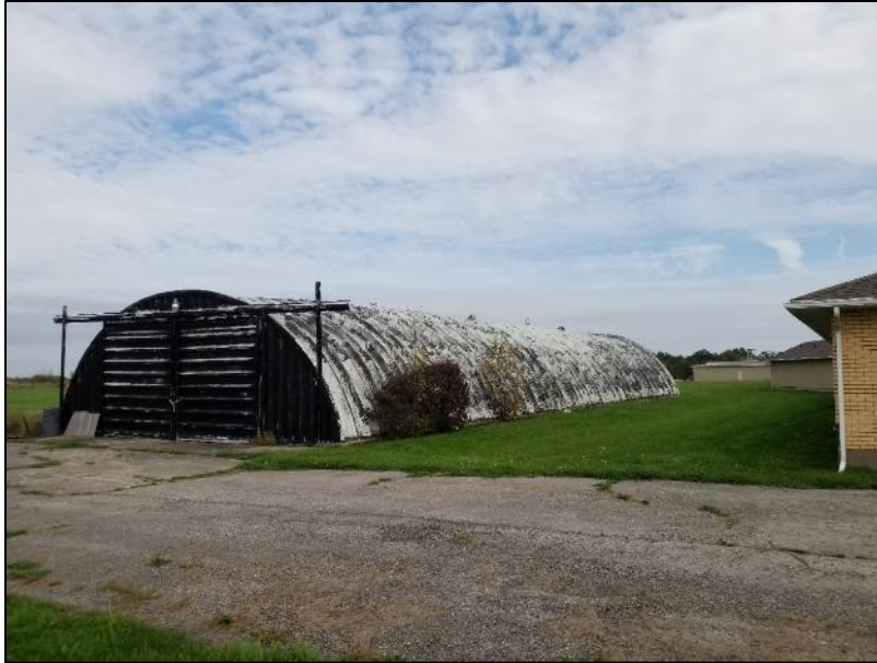
Image 7: View of metal shed within study area.
