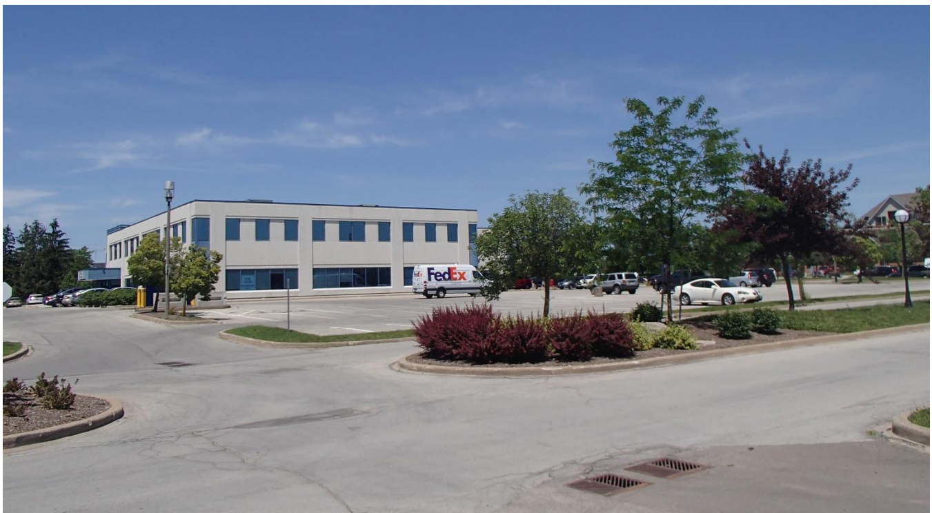
Looking north across parking lot and two storey office building off of Schmon Parkway.
