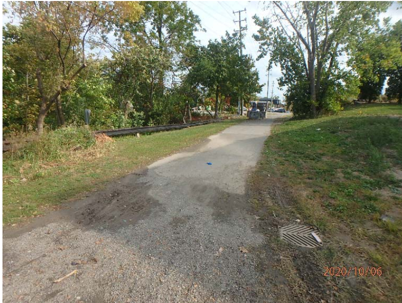
Photograph No. 1: 0013: Roadway over the structure looking east.
