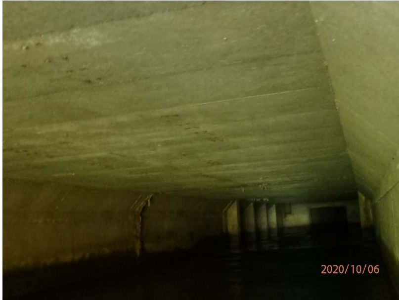
Photograph No. 3: 0065: Interior of structure looking south.
