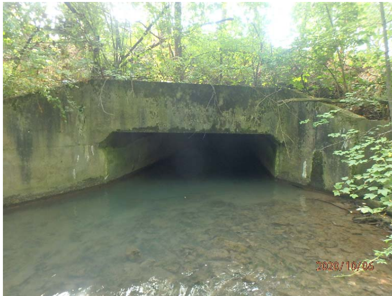
Photograph No. 2: 0033: North elevation.
