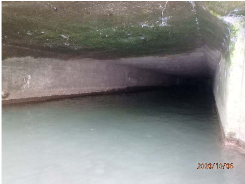
Photograph No. 4: 0037: Interior of structure looking south.
